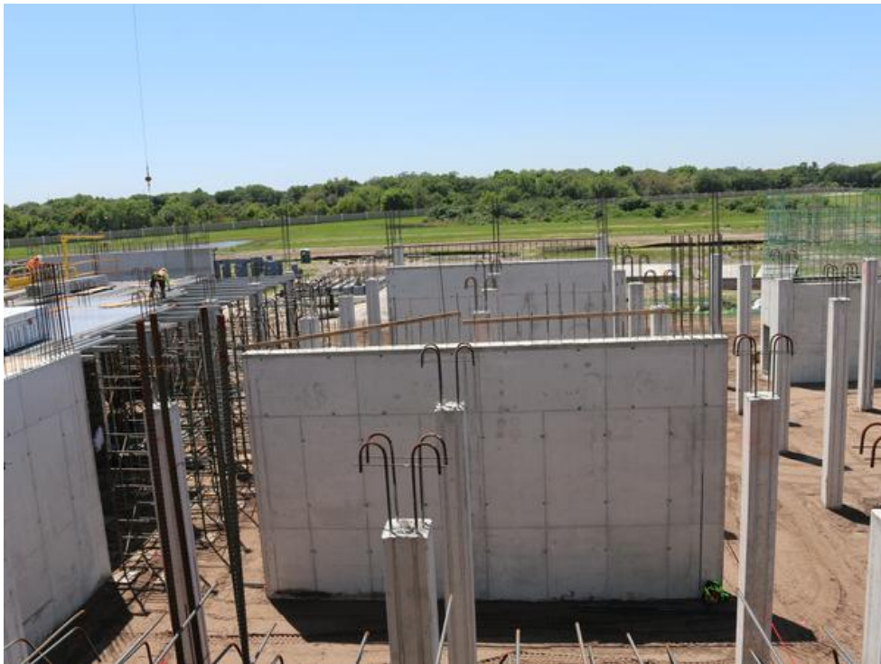
Here's an overview of the Class 1,000 clean room. Matthew Richardson
