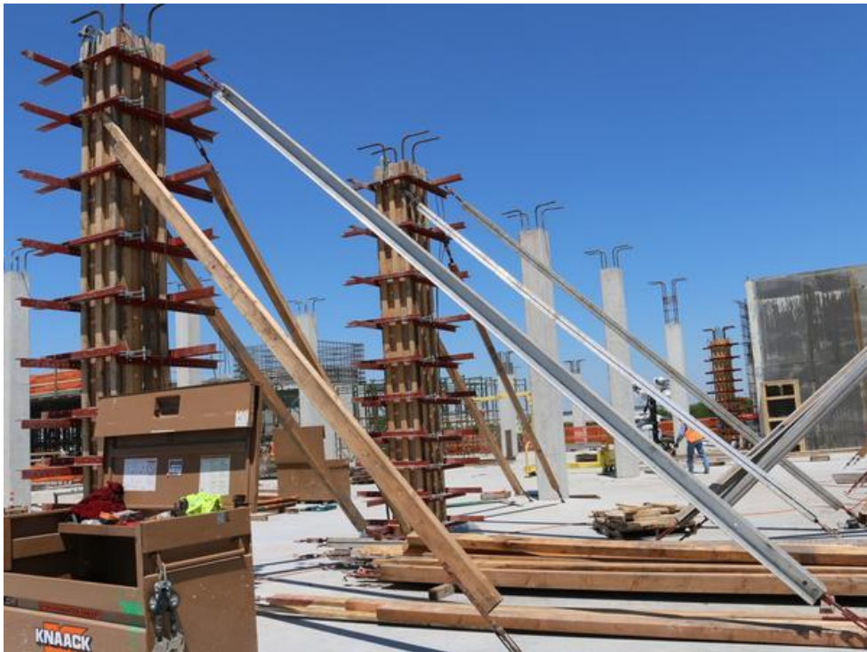
Here's a closer look at the casting method for the concrete pillars. Cement is poured in, dried and then the cast is removed. Matthew Richardson
